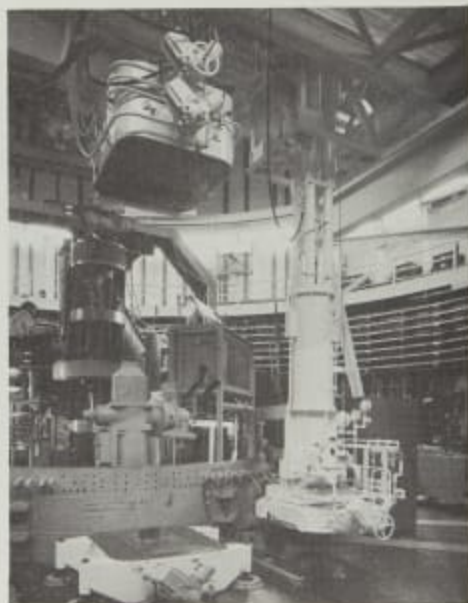
View inside the reactor building showing the fuel handling machine in the foreground and the above-the-plug reactor mechanisms in the background.
