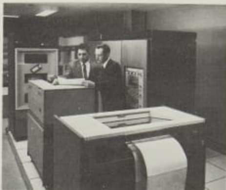
A malfunction detection analyzer was designed and installed on the Fermi I reactor. Composed primarily of an IBM 1800 computer, the system monitors reactor operation for reactivity balance, subassembly outlet temperature rise, and fission product detector response.
